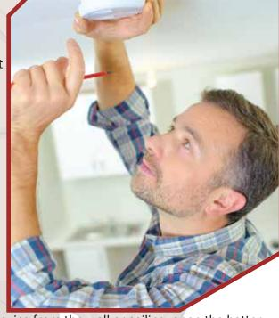
battery is to remove the device from the wall or ceiling, open the battery compartment, pull out the old battery, and put in a new one. Some detectors are connected by cables. These are easily disconnected when you are removing it from the wall and reconnected afterwards.
